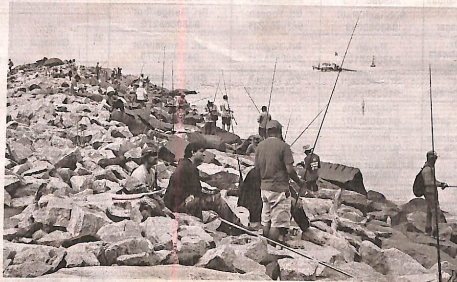
A breakwater in sea at Panambur near New Mangalore Port. ■ FILE PHOTO
