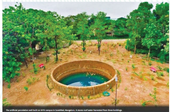
A well collected 12 lakh litres of rainwater this June-July
