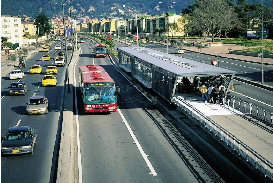
Figure 1.5 Closed BRT System – Bogota BRTS (Source: Google Images)
