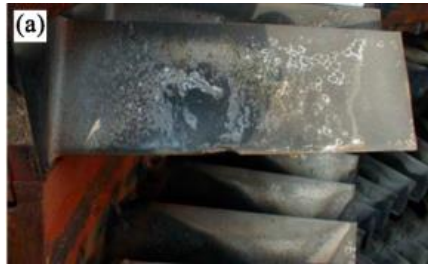
Figure 1.3 Erosion on leading edge of a turbine fan blade (Alqallaf et al. 2020)
