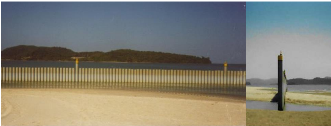
Figure 1.2 Front and side view of a single row pile breakwater constructed at Pelangi beach resort, Langkawi, Malaysia (Reedijk and Muttray 2009)
